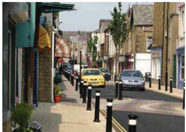
Yorkshire Street improvements
